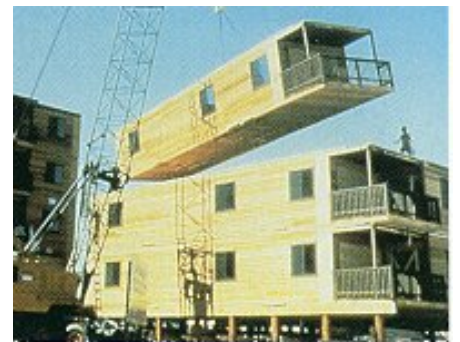
Modular Apartments being craned into place.
