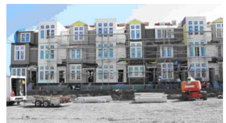
Modular Apartments being craned into place.
